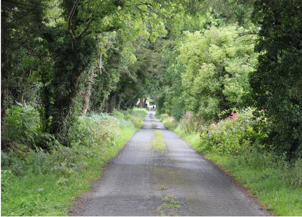
Current view – Link to Kilderry Lane, Muff
